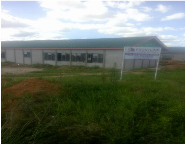
building OF cLASSROOM BLOCKS AT RUWA
